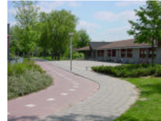
Separate infrastructure for cyclists and pedestrians near the school. Cars move on distance and biking becomes safer and faster!
